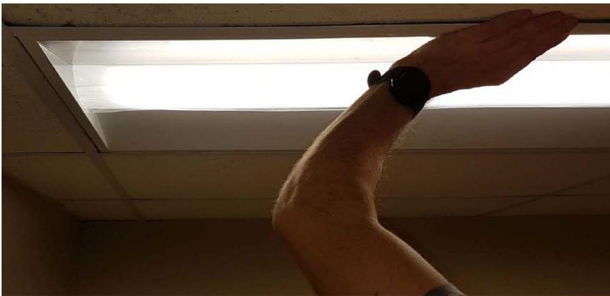
7b. For ceilings with 1/2" T-Grid, install the second L-Bracket as the TDK rotates into place. Then secure it with (2) sheet metal screws (not provided).
