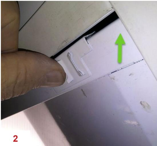
2. Push the fixture back into the grid holding both C-Clips in place.
