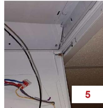
6. After the top left and top right hinge bolt HEADS have been installed into the LIFT RAIL slots, the fixture body may be allowed to hang for hands free splicing. Install the safety cable provided at both ends of the fixture prior to splicing. Proceed with wire splicing with ground wires being spliced first. Use the power disconnect provided for line and neutral (6a). For new construction, replace the cover plate with knockouts (6b).
