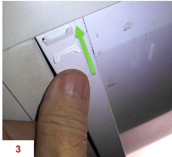
3. Slide both C-Clips toward the end of the fixture assuring good contact with the ceiling grid.
